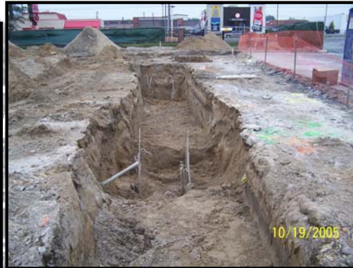
Trench Excavation for Grade Beam
