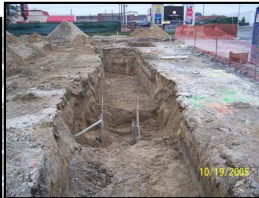
Trench Excavation for Grade Beam
